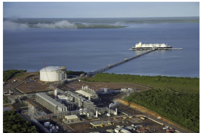
Figure 2. Aerial view of the 3.7 MTPA Darwin LNG plant– the world’s first liquefaction facility to use high efficiency aeroderivative engines. The 188,000 m 3 storage tank and the 1350-meter jetty and loading dock can also be seen.
