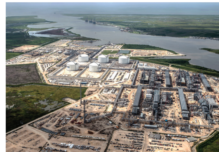
Sabine Pass Liquefaction — Five LNG trains in construction
